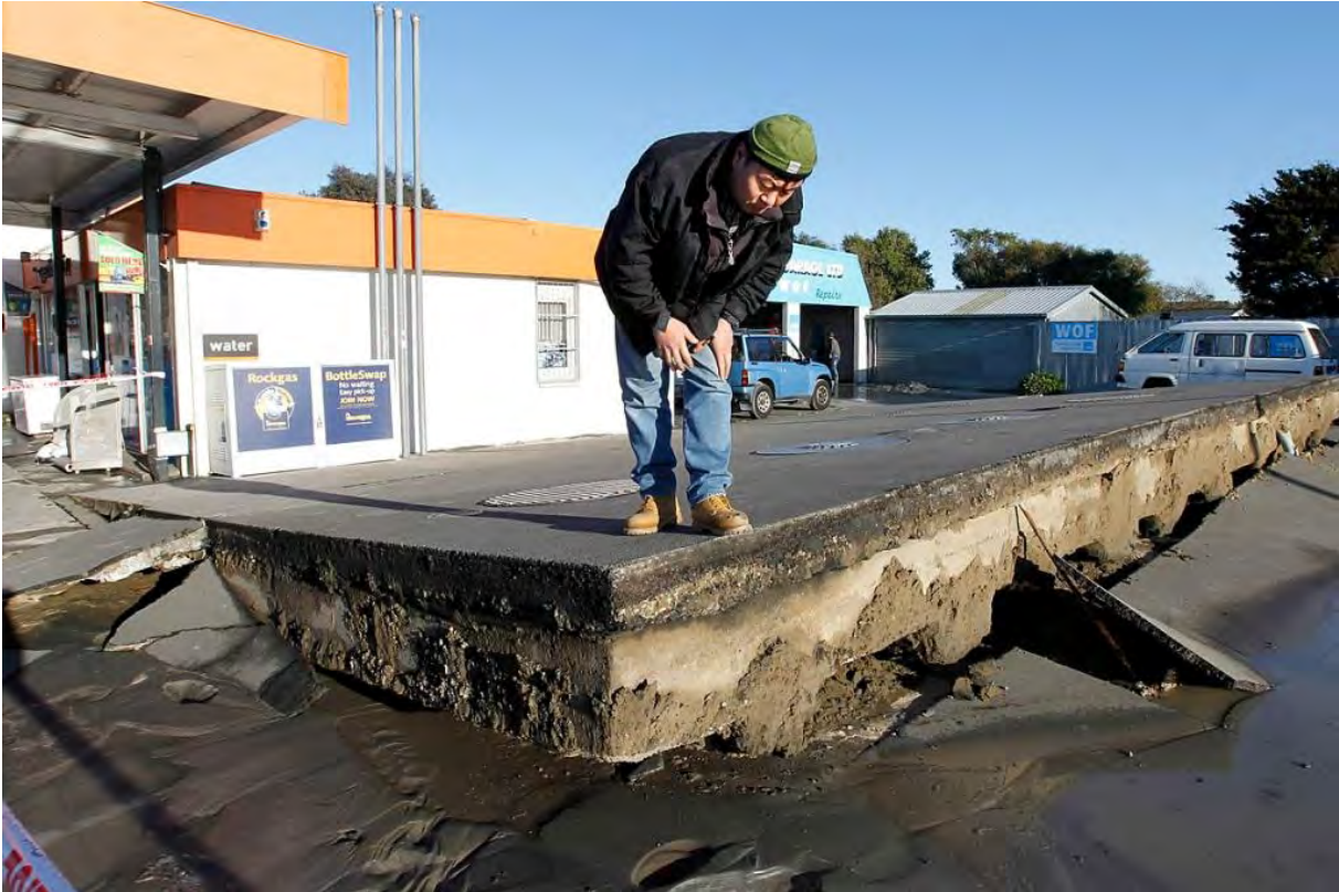
Figure 6 Fuel tanks have buoyed up through the ground surface as a result of liquefaction of the enclosing sediment, .Christchurch area, February 2011. Photo: R.D. Beetham, GNS Science.
