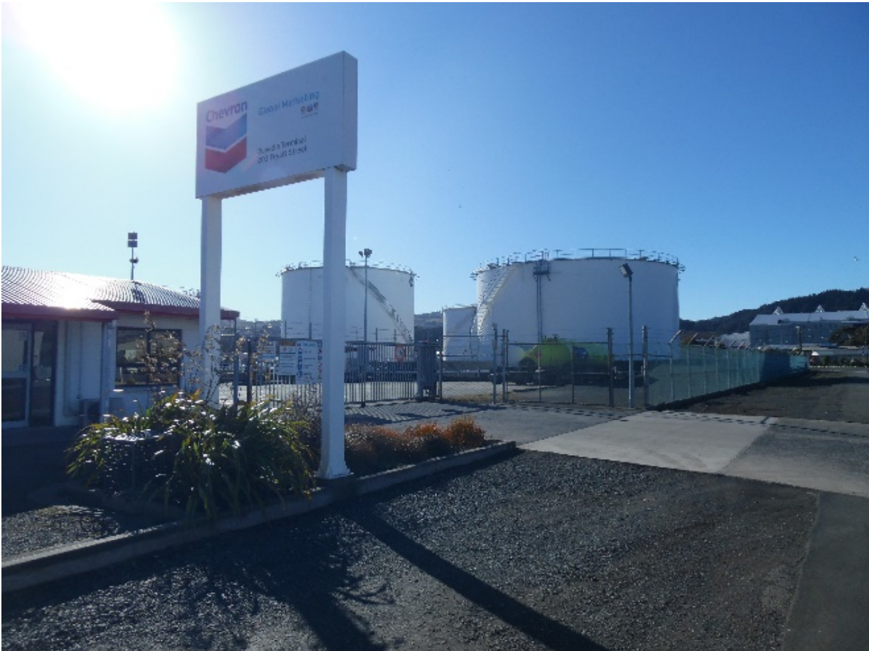
Chevron's Fuel Terminal
